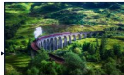
Glenfinnan Viaduct, Inverness-shire, Scot-
